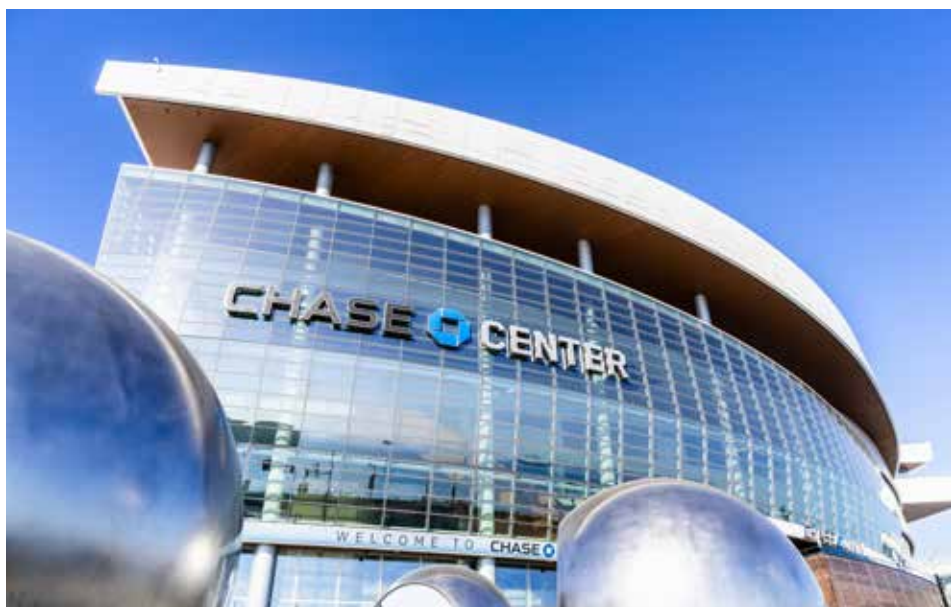
The Chase Center in San Francisco has more than 250 Wi-Fi 6E access points.
